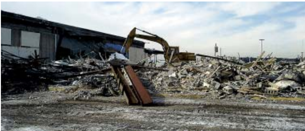
Demolition at Hills and Dales shopping center.
