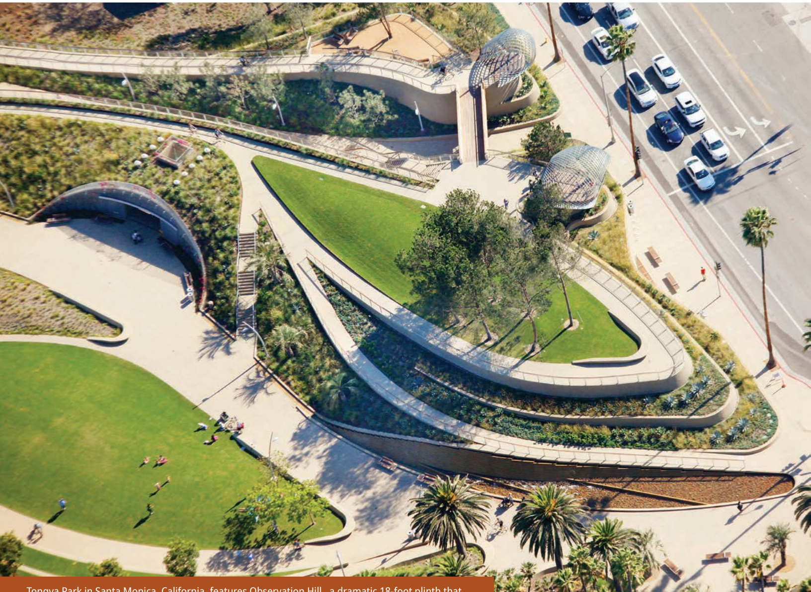
Tongva Park in Santa Monica, California, features Observation Hill, a dramatic 18-foot plinth that offers views of the surrounding beach area and buffers noise from the street. Ramps make the hill and the park accessible to all. Photo by Tim Street-Porter, courtesy of James Corner Field Operations.
